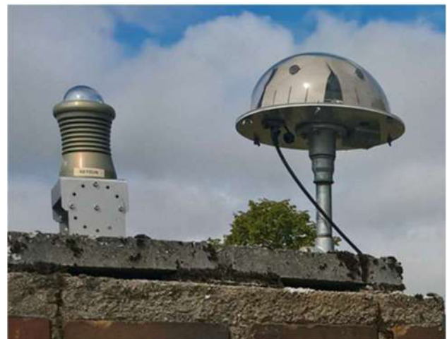
Figure 2 – DEBB01 and AMS16 mounted side-by-side at a roof-top in Ketzür.
